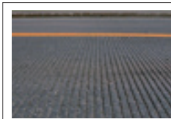
Grooving, whereby grooves are carved on the road surface, helps prevent traffic accidents by alerting raptors of approaching vehicles through the sound generated by vehicles running over the grooves.
